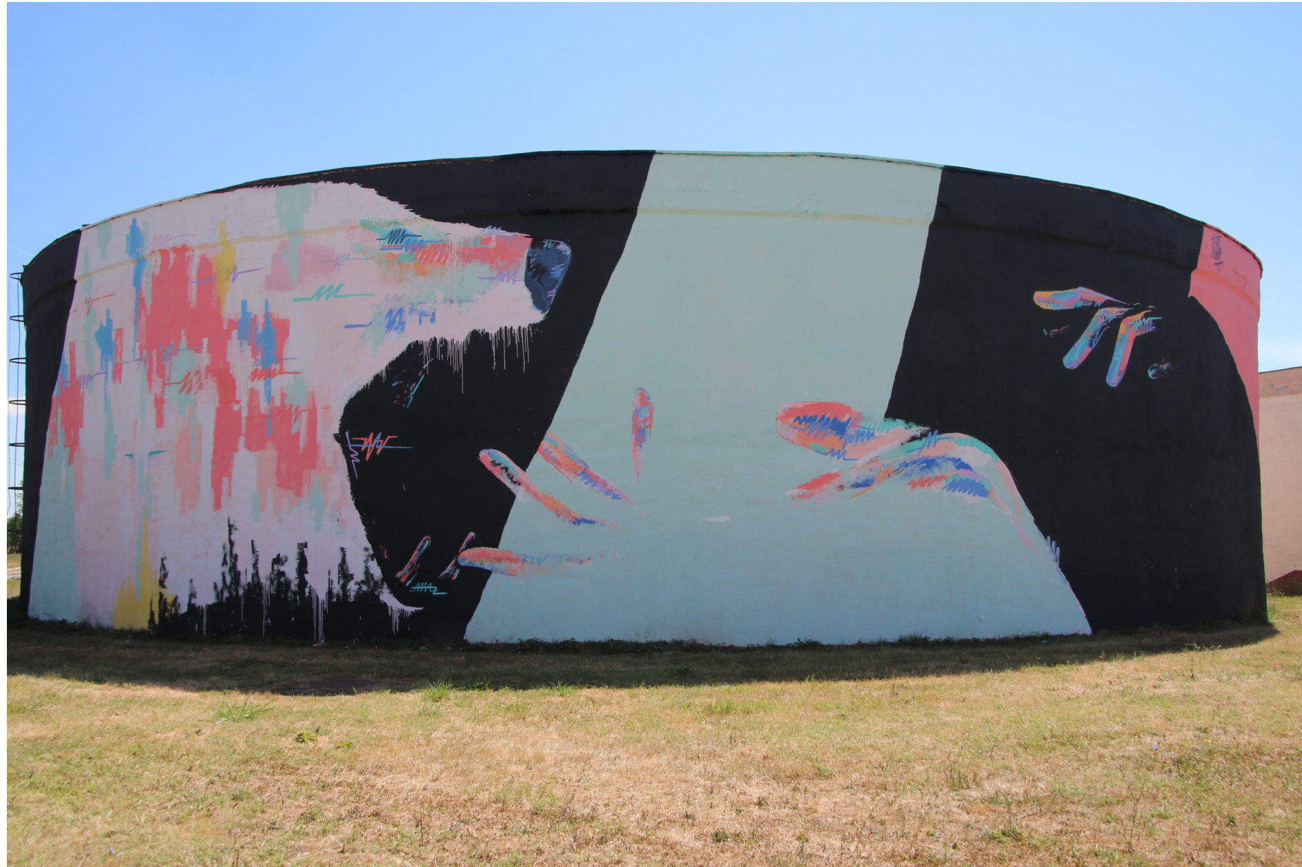
FISART 2017 – Txemy / Spain - Cylindrical Drinking Water Tank with a diameter of 30m at AQUATIM
